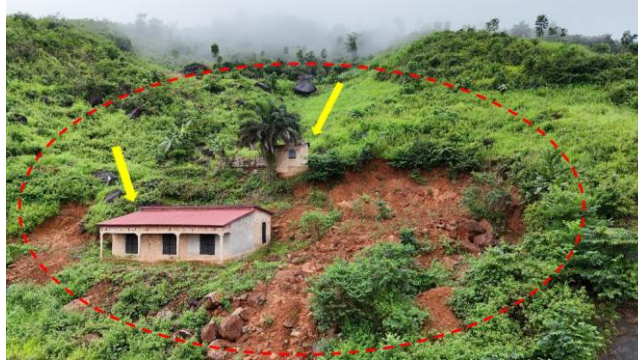
Figure 6. Construction on unstable slopes
